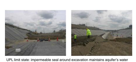
UPL limit state: impermeable seal around excavation maintains aquifer's water level. Weight of fill selected using EC7's principle of 'characteristic' value
